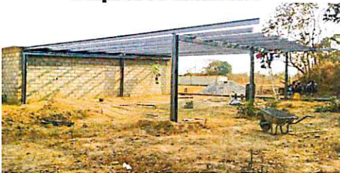
Bible College room addition
